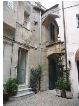
Figure 10 – The curve shaped masonry of the Furnaxin “intermittent kilns” in the historical centre of Cogoleto
